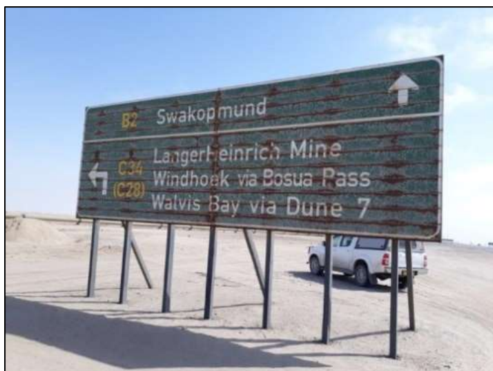
Figure 7: Corroded Sign on B2 Road
